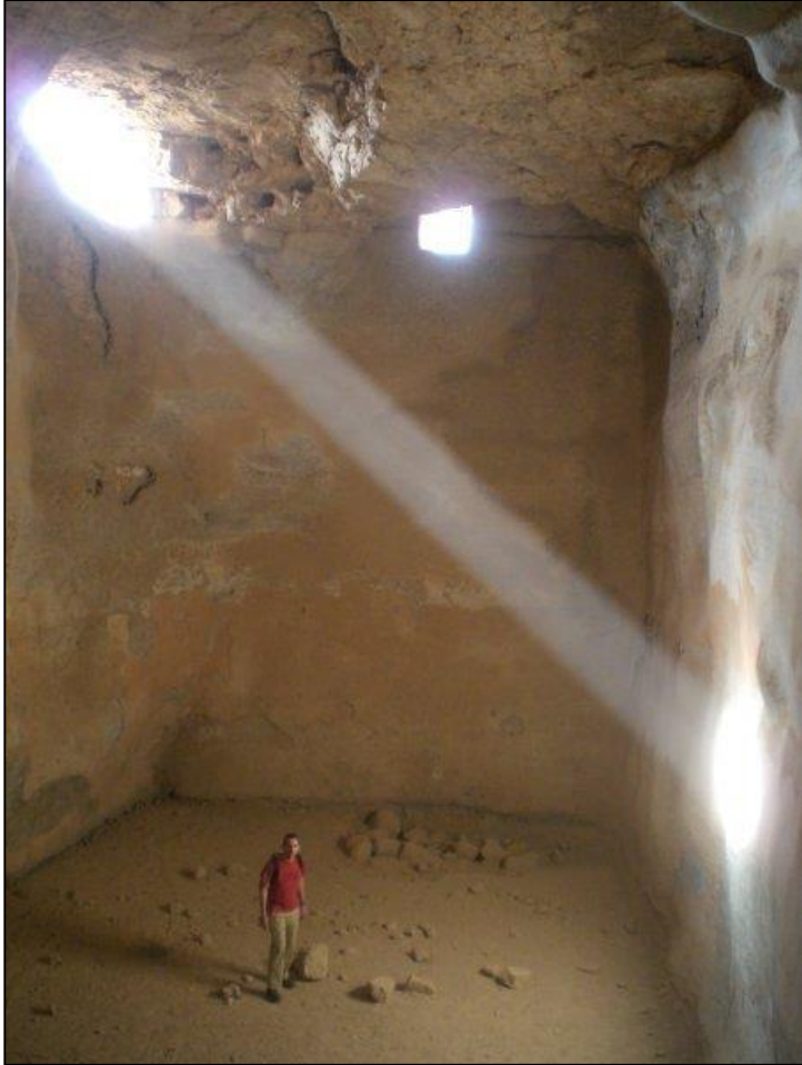
One of several water cisterns on Masada – carved out of mountain and lined w/ waterproof plaster
